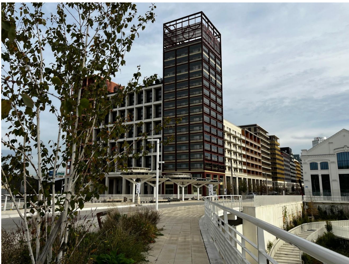
Photo: 24 Residential buildings and riverside promenade in the Saint-Ouen sector of the Paris 2024 Olympic Village (ZAC Village Olympique) along the Seine.(Lawson, 2025)
