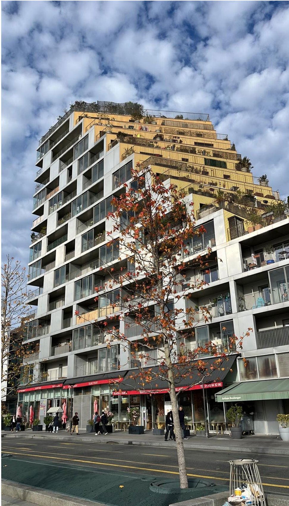
Photo: 20 Residential building with stepped timber terraces, Avenue de France, ZAC Paris Rive Gauche (Tolbiac sector), 13 e arrondissement, Paris (Lawson, 2025)
