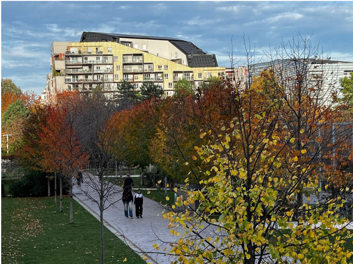
Photo: 23Parc Clichy-Batignolles – Innovative housing surrounding Martin Luther King in the Clichy-Batignolles eco-district (17 e arrondissement, Paris).
