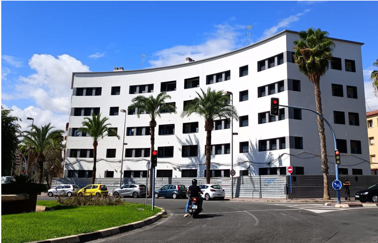
Photo: 27 Newly constructed public rental housing in Valencia Source: Generalitat Valenciana (2025)
